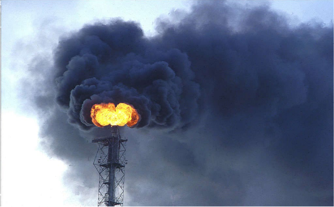
Flare stack at oil refinery in Immingham, UK © Les Gibbon / Greenpeace
